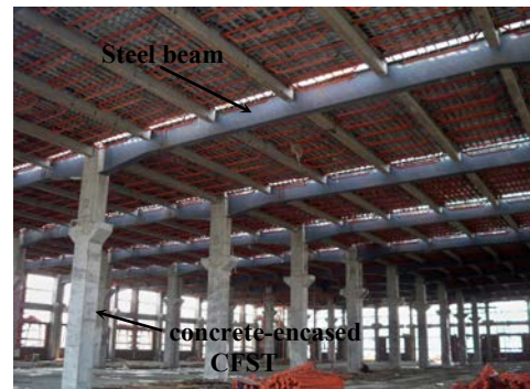
(b) Concrete-encased CFST column to steel beam
