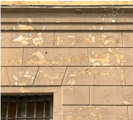
Craquelado (RF7) Crackling (RF7)
