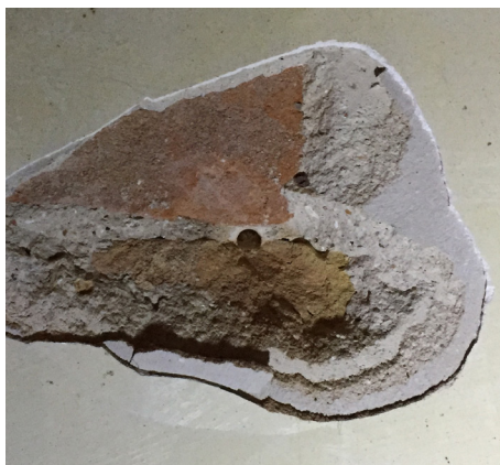
Perforación del revoco (RF5) Plaster perforation (RF5)
